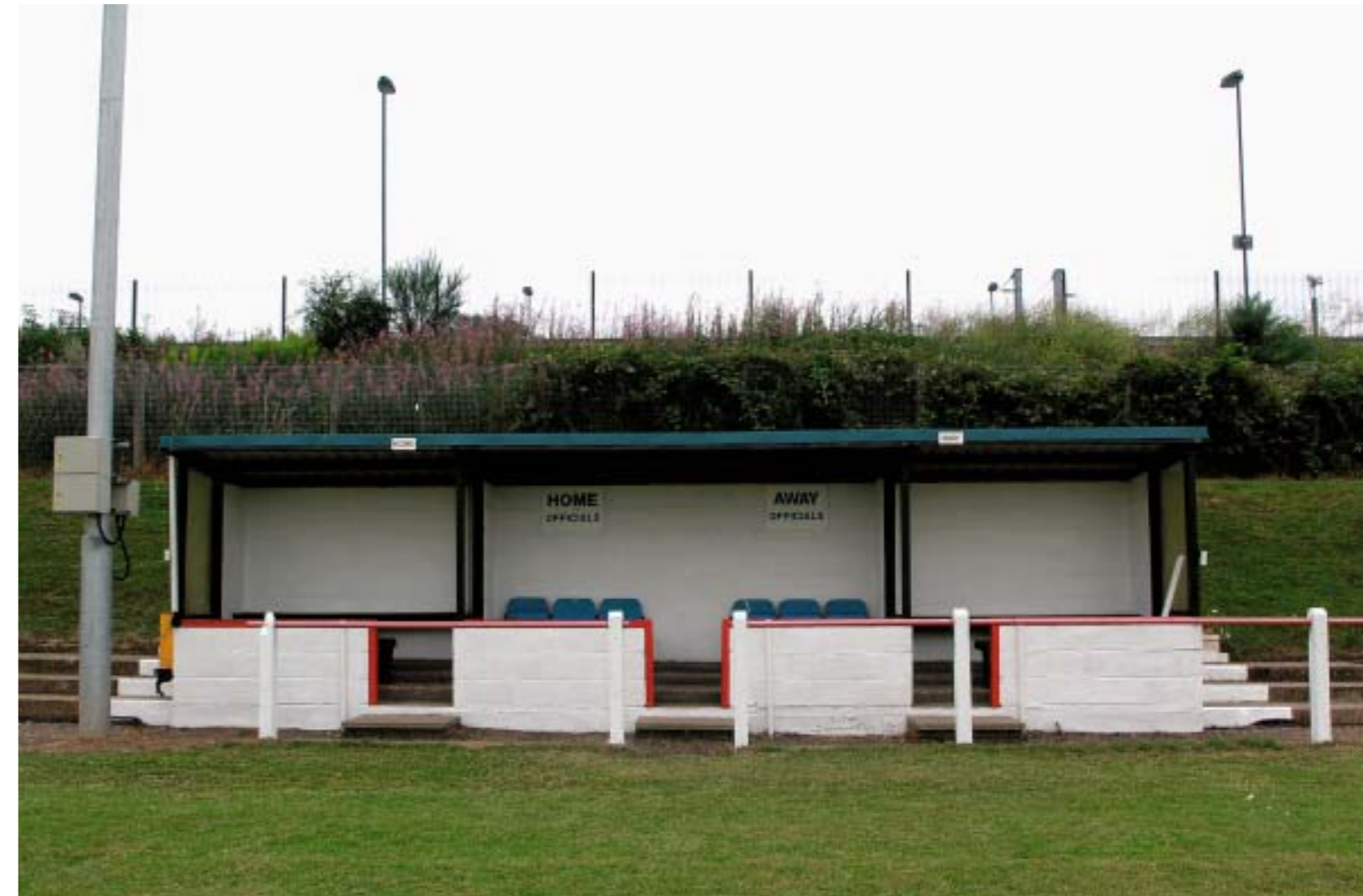
Pilkington XXX FC (Midland Combination League) Triplex Sports, Eckersall Road, King's Norton, Birmingham
